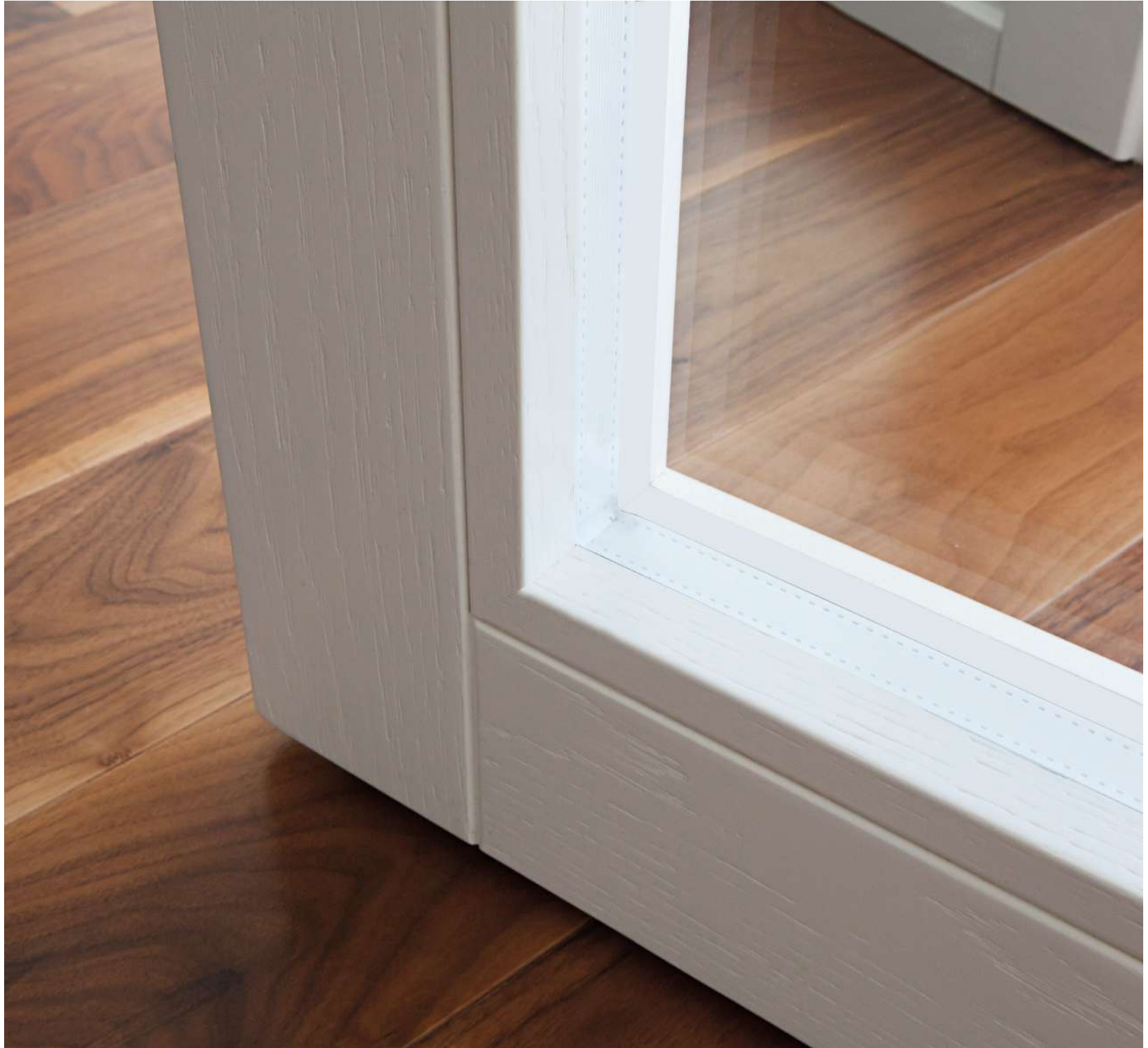
Particolare fermavetro Legno Design in rovere lamellare spazzolato - finitura laccata RAL 9010 - 5 Gloss Galss - holder design detail - brushed laminated oak - painted finish Ral 9010 - 5 Gloss
