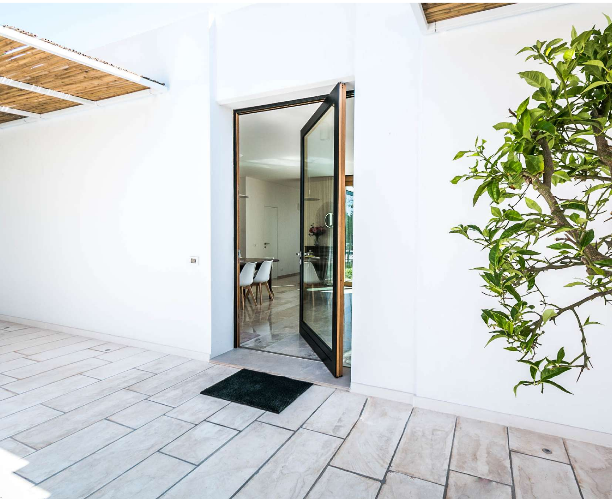
Portafinestra con cerniere a bilico verticale FritsJurgens (portata 500 Kg) French door with FritsJurgens vertical pivot hinges (capacity 500 Kg)
